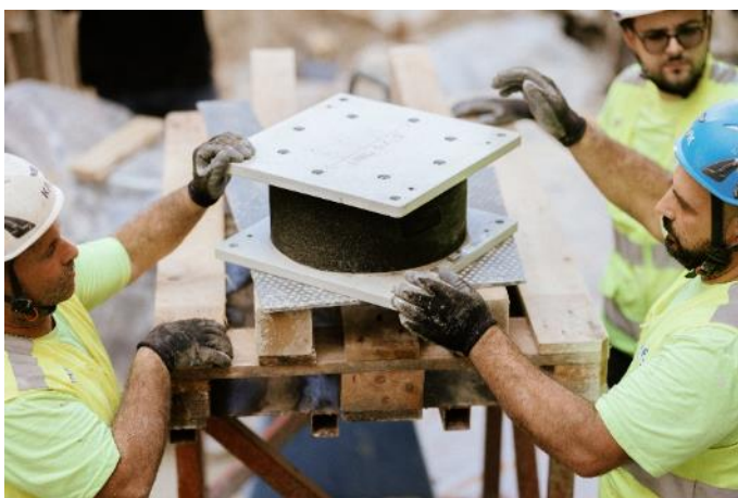
Fig.2 – Isolatore HDBR (High Damping Rubber Bearing)
